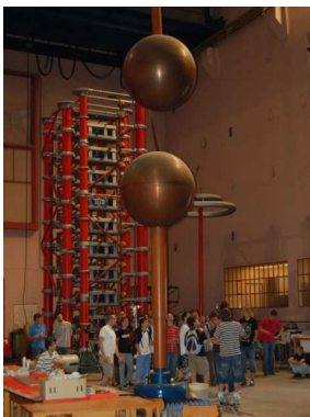
Figure 4. High voltage laboratory at Slovak University of Technology in Bratislava
